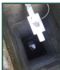
After sewer cleanse, shown by drop in graph
