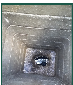
Blockage in sewer shown by peak in graph
